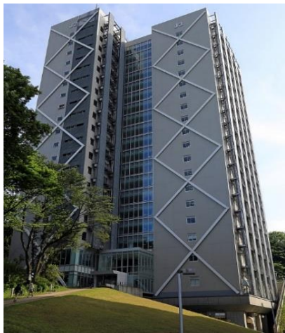
Fig.1 Photo of J2-3 building
