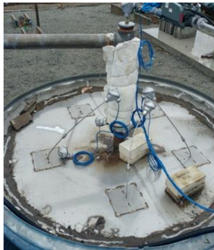
Fig. 2.2 Heat storage system tank
