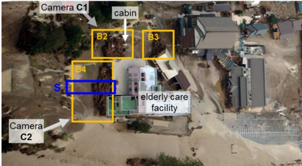
Figure 4.24: On-site photo of the same area after the disaster.
