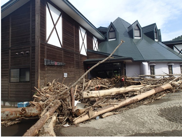
Figure 1.1: The damage of driftwood to structures.
