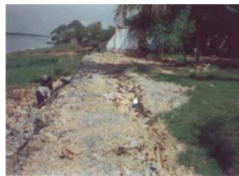
Fig.1a Gabion retaining wall
