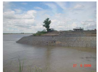
Fig.4f Man-made slope rehabilitation
