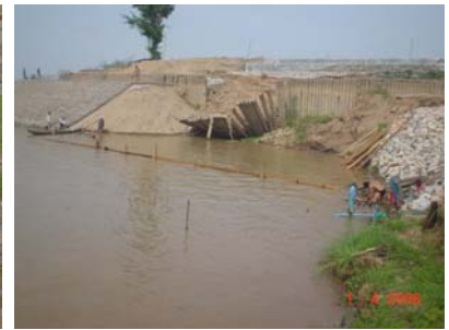
Fig.4d Slope rehabilitation works
