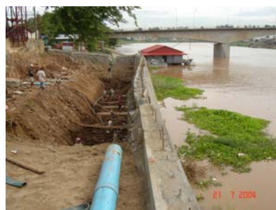
Fig.3a Retaining structure
