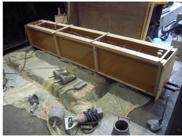
(c) Formwork for SF30-10-r30-L
