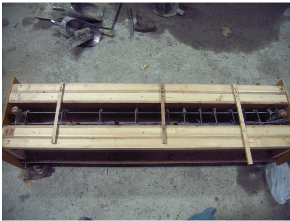
(b) Formwork for SF30-10-r32-S
