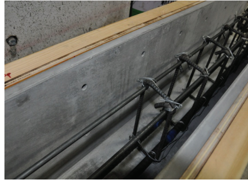
Installing reinforcement bars
