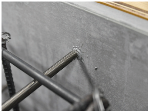
Installing the screws and bolts
