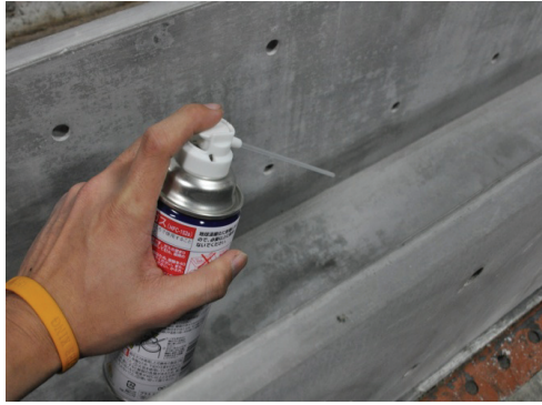
Cleaning of permanent formwork
