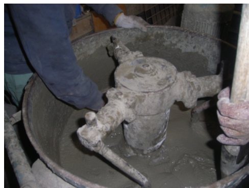
Mixing of concrete
