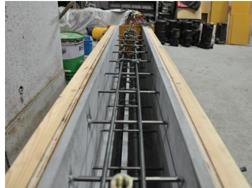
Specimen with ready for casting
