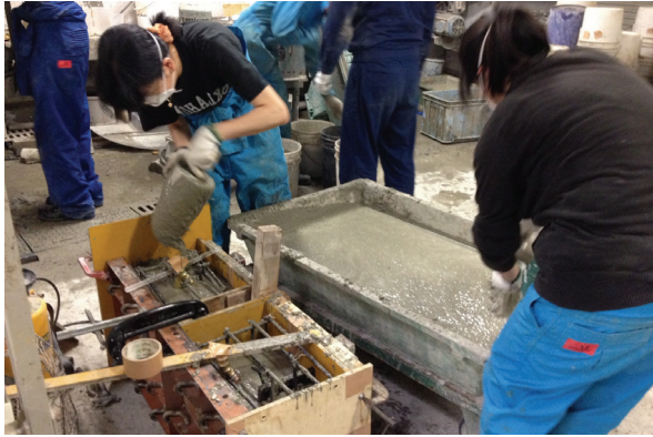
(f) Casting of concrete
