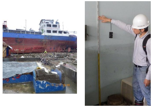
Fig. 11. (Left) Homes demolished by drifting ships near Tacloban Harbor. (Right) Typical soiling inland in downtown Tacloban, where only surge (no waves) was present.
