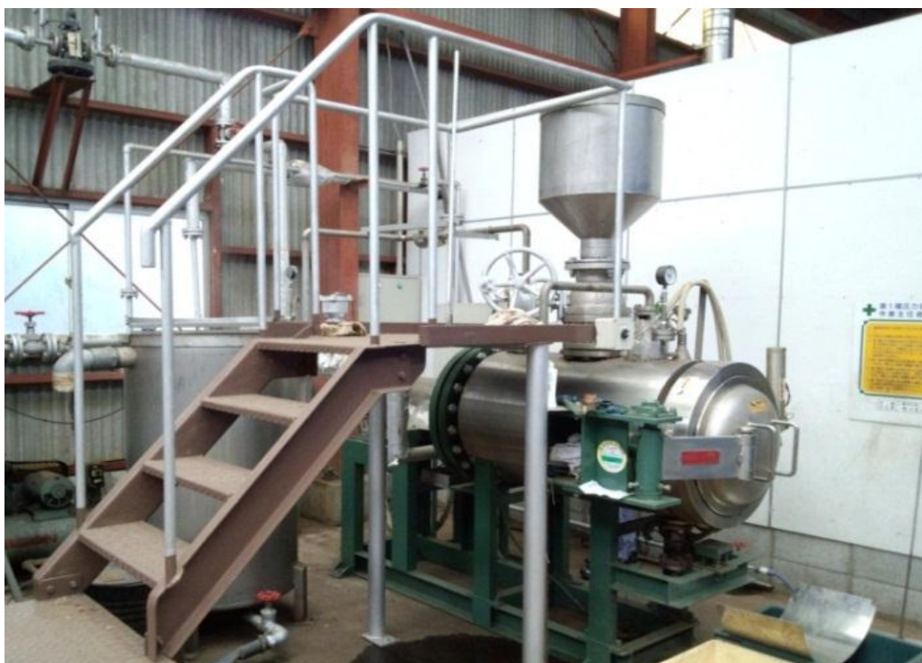
Fig.4.2. Snapshot of the HTT facility
