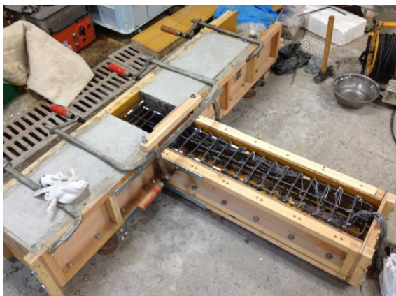
(e) Setup formwork for PP-ECC.
