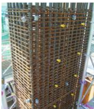
Photo 1.1.4 Large amount of longitudinal and shear rebars in bridge column.
