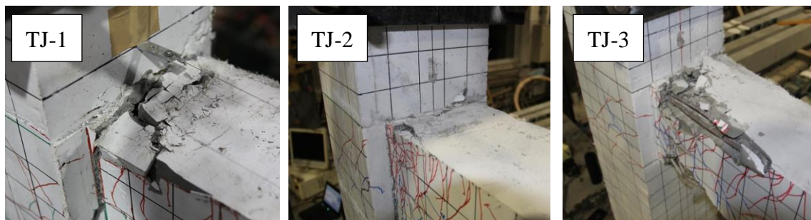
Photo 5.4.3 Damage at the top of the beam by the end of tests.
