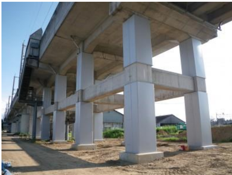
Photo 1.1.1 Rigid-framed railway bridge.
