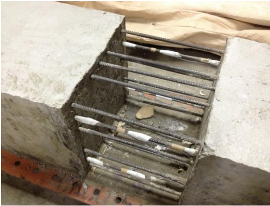
(b) After removal of temporary formwork.
