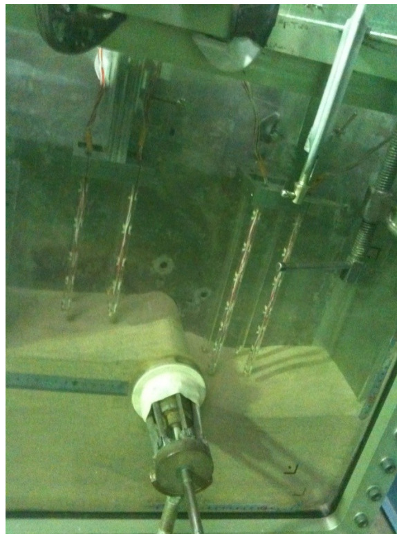
Figure 3.46 Installation of pile groups
