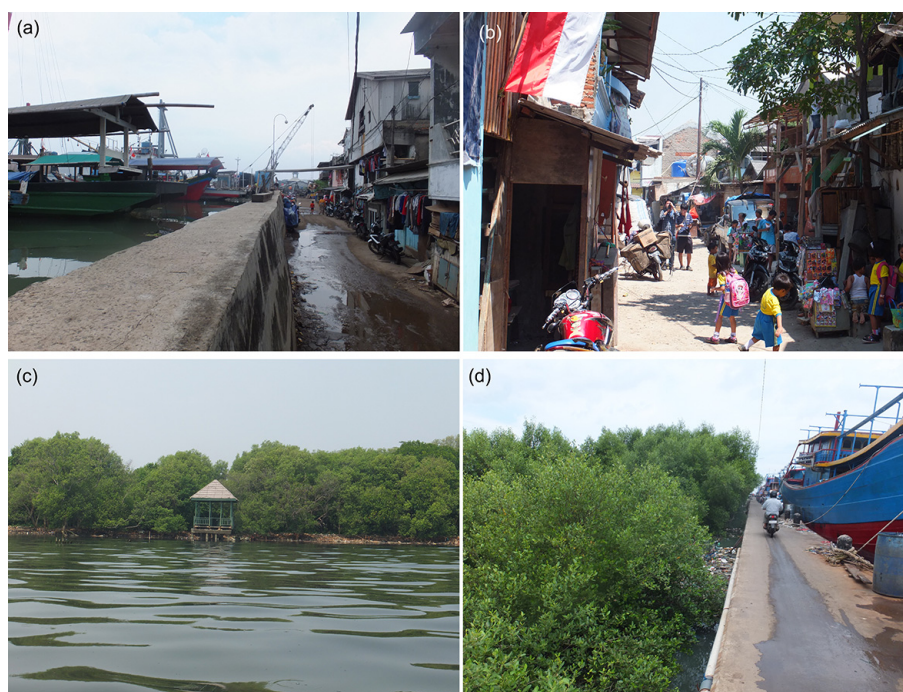
Figure 2. Coastal areas around Jakarta (photos taken by the authors during field surveys in the period between May 2015 and February 2016). (a) A thin coastal dyke protecting a community experiencing rapid subsidence (district of Pluit, northern Jakarta). Leakage of seawater through a concrete joint was observed during the authors' visual inspection on 6 February 2016. The sea level was 1.3 m higher than the road. (b) The town centre of Pluit, with a high population density and long narrow paths. (c) Mangrove conservation site in Jakarta (see Fig. 3 for its location) (d) Mangrove rehabilitation site in the Jakarta Fishing Port (see Fig. 3 for its location). The mangrove belt is around 20 m thick and can effectively protect the port basin from wind waves.
