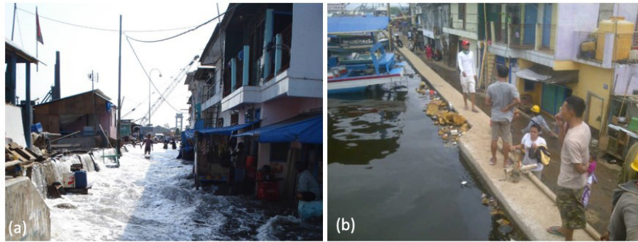
Figure 5. The district of Pluit in Jakarta is situated below sea level. The area suffered extensive inundation during high tide on 26 November 2007 (left). The thin dyke protecting the settlement was raised by about a metre after the 2007 high-tide event by the local government, obstructing people’s view of the sea. The photo was taken on 18 October 2013 (right). (Photos: courtesy of Brinkman, J. J., Deltares).
