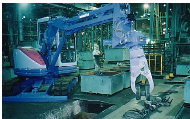
(a) Handling in foundry
