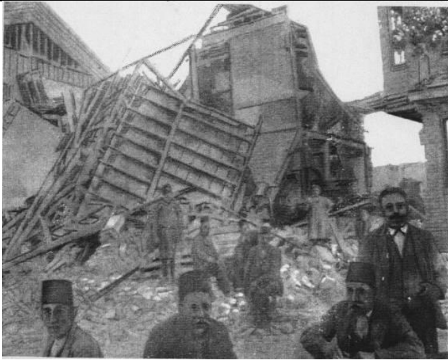
(e) Collapsed buildings at Sarkoy (Sadi, 1912).
