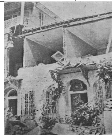
(h) Damaged building at Canakkale (Sadi, 1912).
