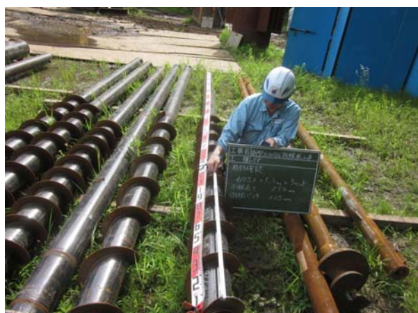
Photo 5.1 Continuous helical pile
