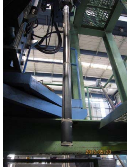
Photo 4.2 Straight sided pile
