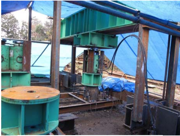
Photo 3.7 Loading tests (W6A-C)
