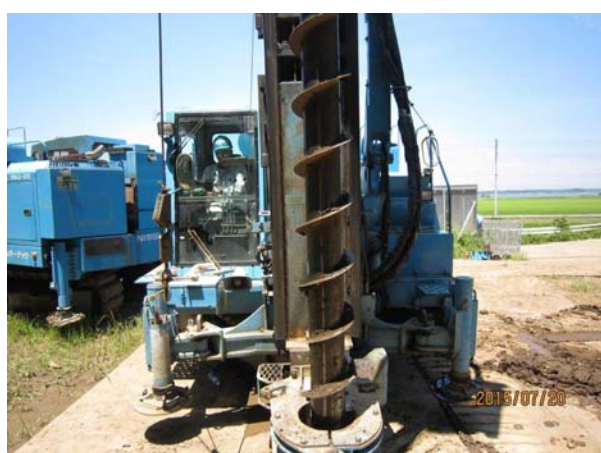
Photo 5.3 Continuous helical pile
