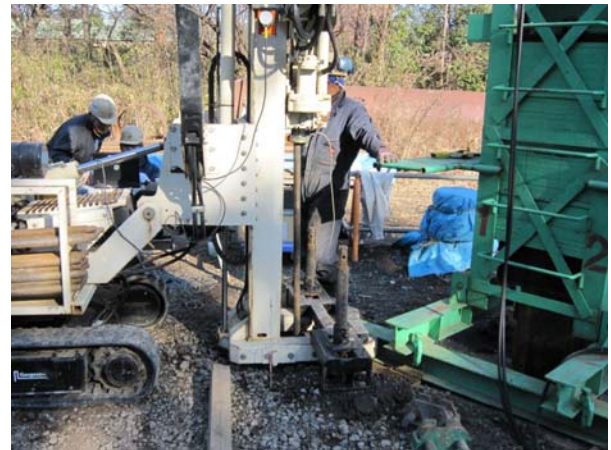
Photo 3.2 Cone penetration test
