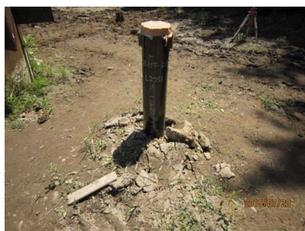
Photo 5.4 After installation (B-MC)
