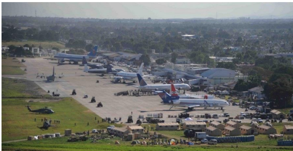
Figure 1-1 Air side congestion in Port-au-Prince airport in Haiti
