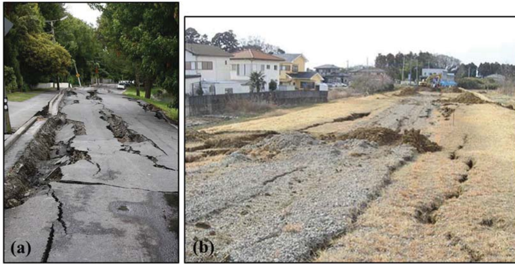
Figure 4.16. Damages induced by lateral spreading; (a) 2011 Christchurch earthquake, (b) 2011 Tohoku earthquake (Towhata, 2011).
