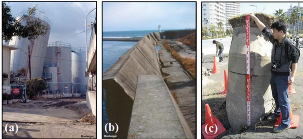
Figure 4.14. Soil liquefaction damages; (a) Tank overturning in 1995 Kobe earthquake (UC Davis website), (b) Quay wall overturning in 1995 Kobe earthquake (UC Davis website), (c) Buried structures flotation in 2011 Tohoku earthquake (Towhata, 2011).
