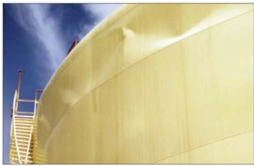
Upper shell of tank suffered damage by sloshing.
