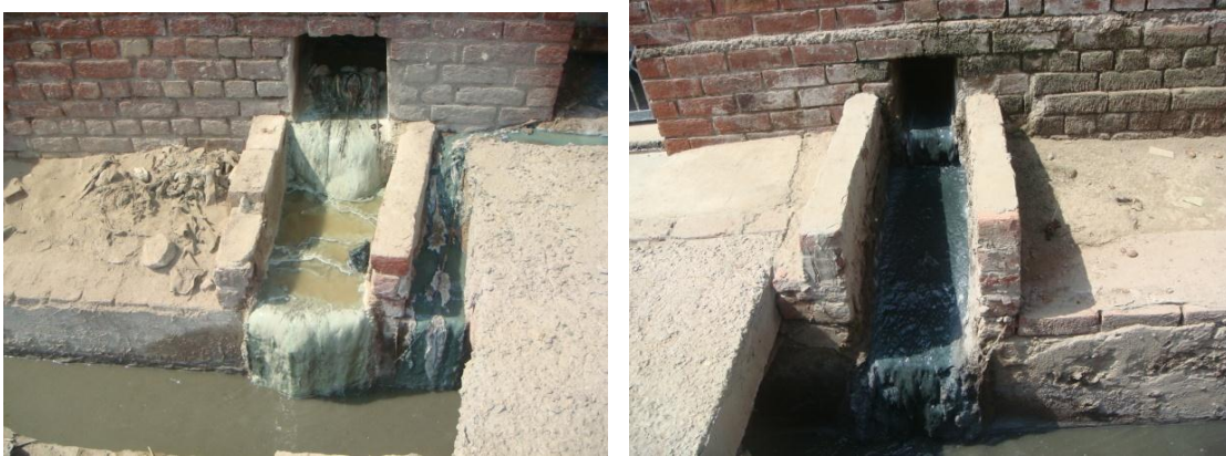
Fig. 4.4: Wastewater containing heavy loads of solid waste (Picture taken in Nov 2008)
