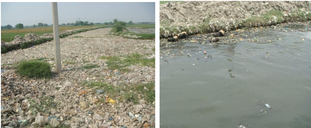
Fig. 4.13: Drain 4 (Drain Rohi) passing through center of Kasur showing the blockage and end of the drain (picture taken in Nov 2008)
