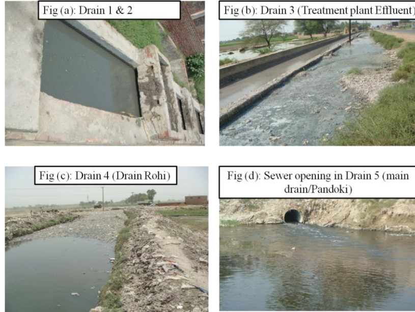
Fig. 2.8: Five drains and underground sewer in Kasur study area (picture taken in 2008)
