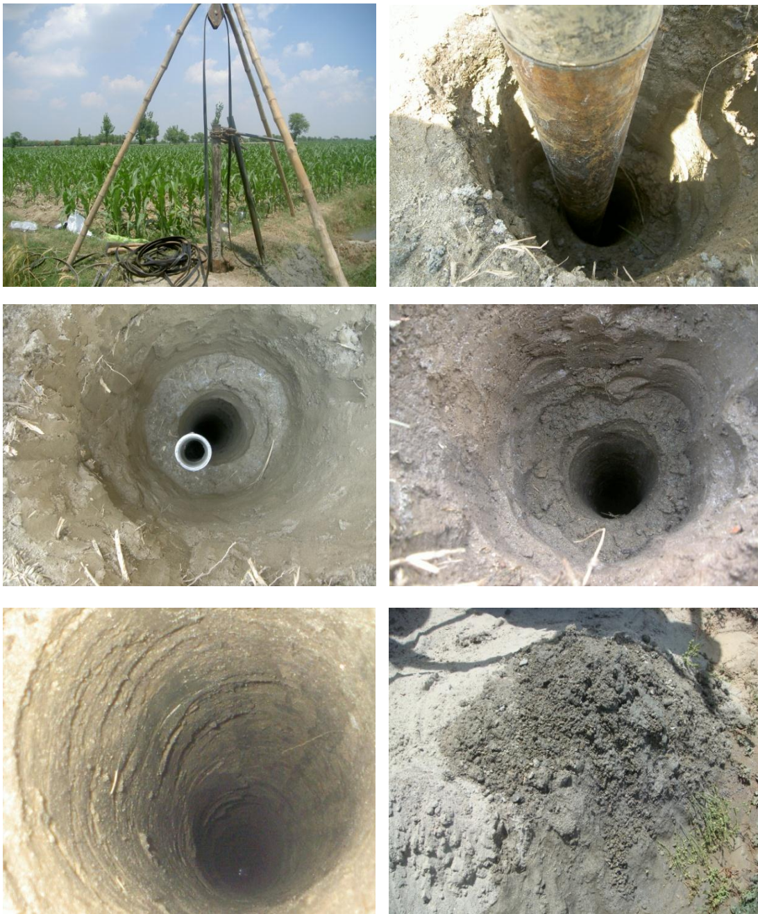
Fig. 4.22: Different procedures, and tools and set up for manual soil bore (April 2011)
