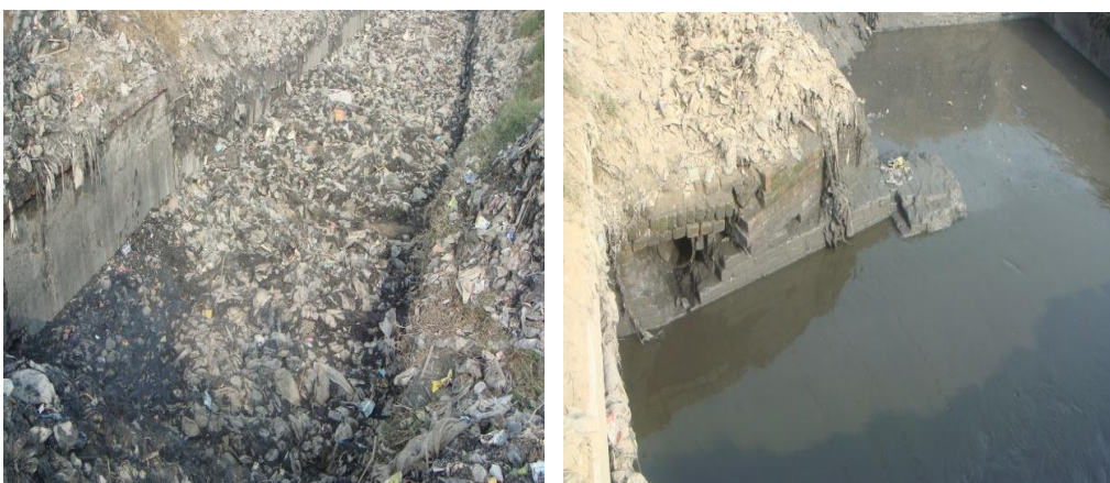
Fig.4.15: Endpoint of Drain 3 into a junction of Drain 3 & 4 (Dec 2009)
