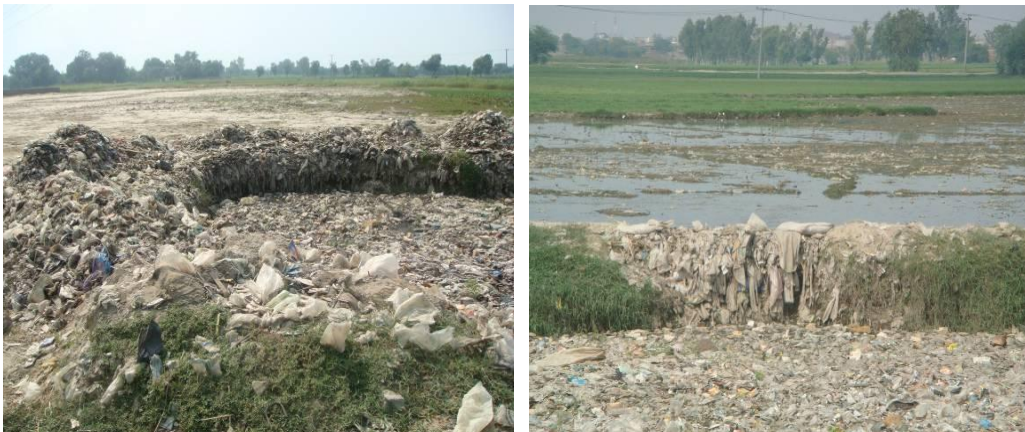
Fig. 4.14: Junction of Drain 3 & 4 completely covered with waste disposal on the sides (picture taken in Nov 2008)
