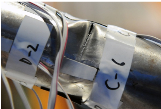
(e) Brace initial crack on the central part (1/33rad-5cycle)
