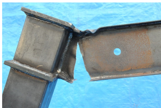
(f) Collapsed specimen after testing
