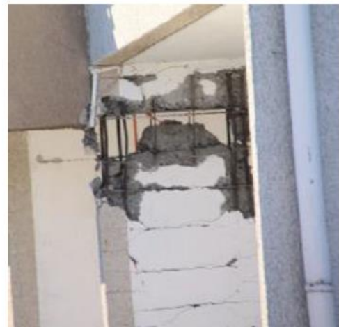
Figure 2.5 - Wall damages with evidence of large tensile strains prior to compressive failures (NEEShub Database)
