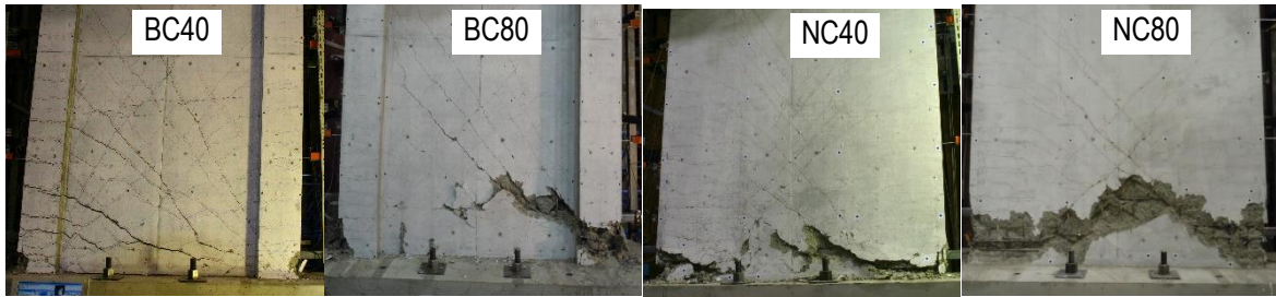
(c) 1.71 shear span-to-wall length ratio walls around peak point
