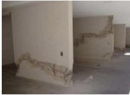
(b) Concrete crushing over wall width
