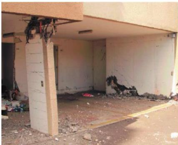
Figure 2.5 - Wall damages with evidence of large tensile strains prior to compressive failures (NEEShub Database)
