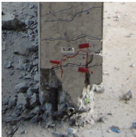
Lower North side
