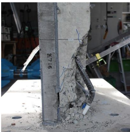
Lower North side
