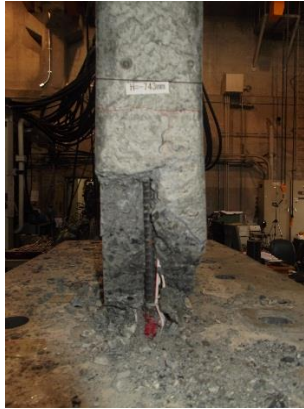
Lower North side
