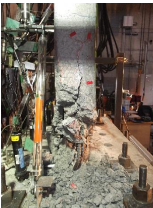
Lower North side
