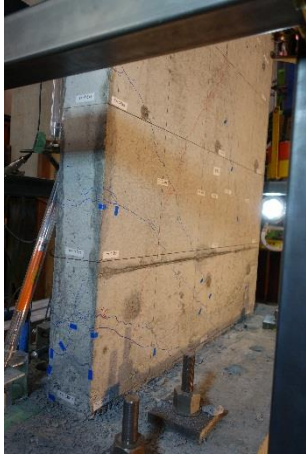
Lower North side
