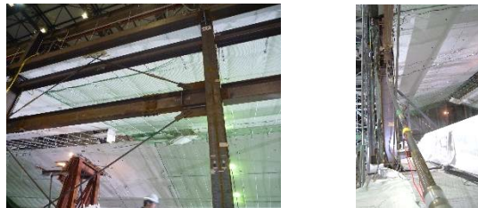
Figure 13: Photograph of wall brace of NC-specimen after No. 17 excitation (Y1 and Y7 side)
