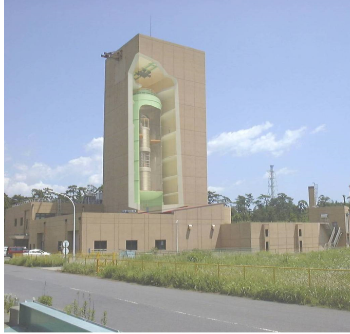
FIGURE 3.1: The JAEA accelerator has been installed inside the building. The photo from JAEA website [3].
