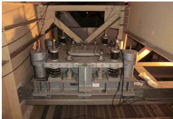
(a) Tuned Mass Damper (TMD)
