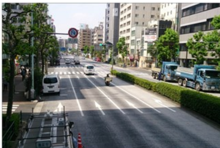
Figure 5-1 Photo from Rx antenna
