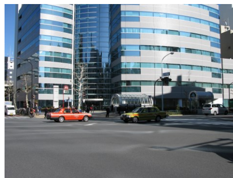
(b) Chamfered shaped building at NLOS2.
