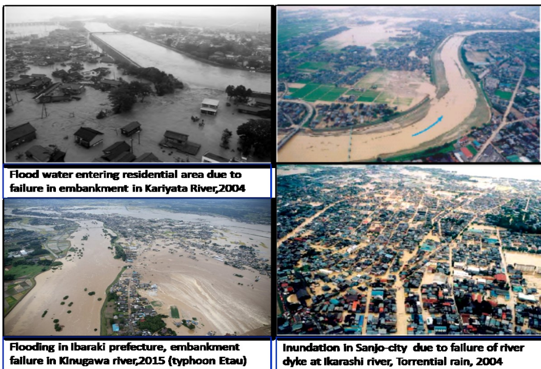
Figure 1.2 Damages caused by the breaching of the levee (Chappell, 2015; Nobuyuki, 2004; Sato et al., 2006)
