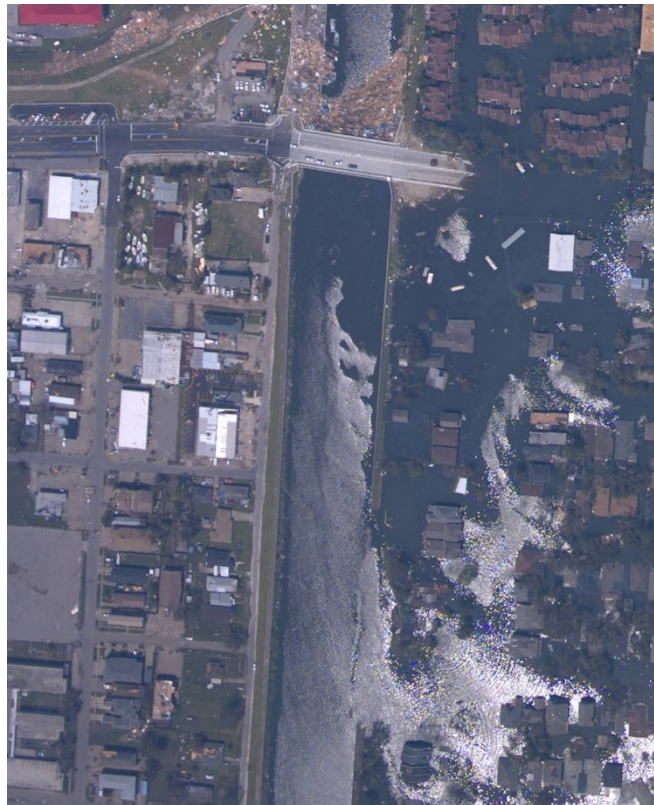
Figure 1.7 Breach in 17 th Street Canal Levee in New Orleans, Louisiana showing inundated neighbourhood ( Bea, 2008)
