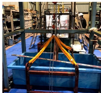
(j) Arrangement of drainage tank
