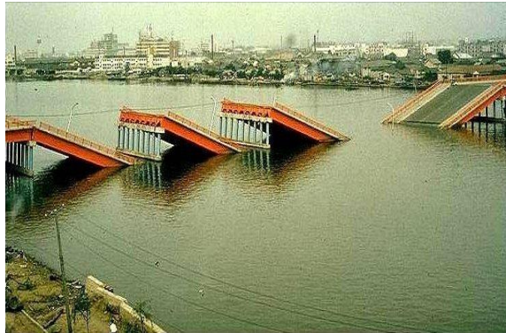
Fig. 1.4. The collapse of the bridge due to liquefaction induced lateral movement of the foundation during the 1964 Niigata Earthquake (Courtesy of the National Information Service for Earthquake Engineering, EERC, University of California, Berkeley, USA)
