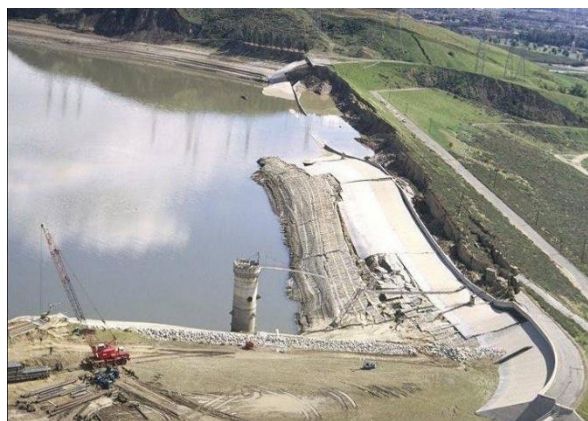
Fig. 1.3. Damage to Lower San Fernando Dam during 1971 San Fernando Earthquake (Courtesy of the National Information Service for Earthquake Engineering, EERC, University
