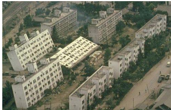
Fig. 1.2. The collapse of buildings due to loss of bearing capacity during the 1964 Niigata Earthquake (Courtesy of the National Information Service for Earthquake Engineering, EERC, University of California, Berkeley, USA)
