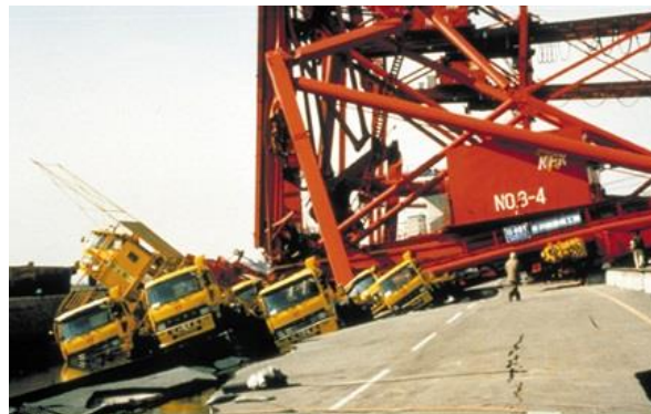
Fig. 1.5. Damage to port facilities during the 1995 Kobe Earthquake (Courtesy of UW College of Engineering, USA)
