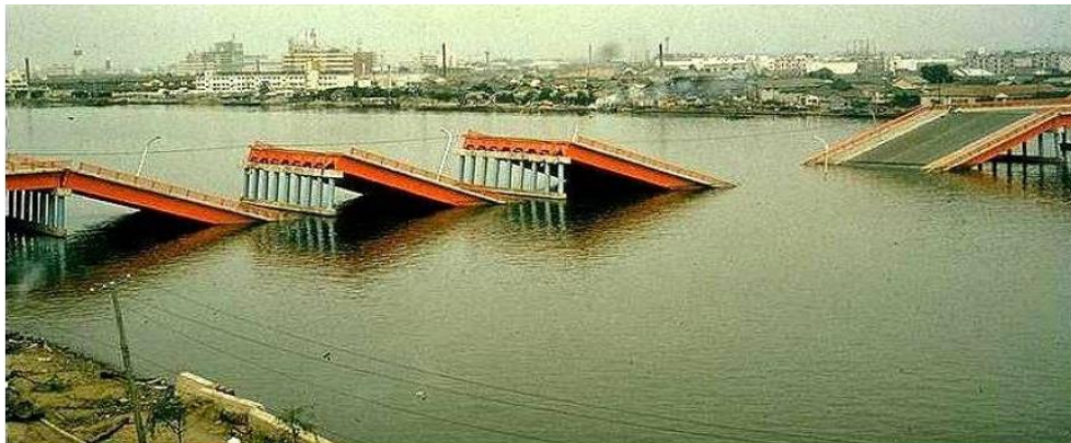
Fig. 1.5: Collapse of Showa Bridge during the 1964 Niigata Earthquake.
