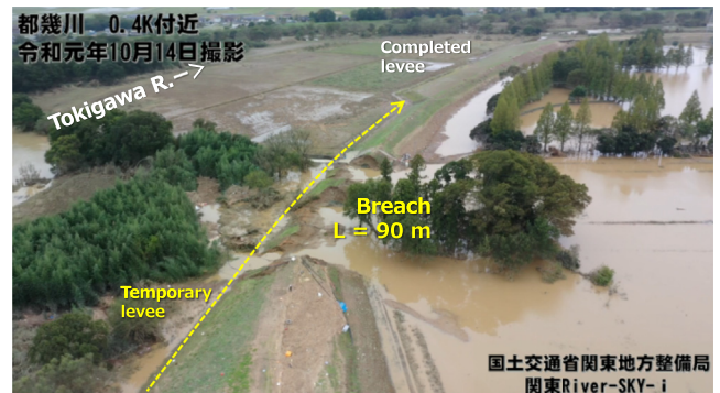
Fig. 7. Breach at 0.4 k on right levee of Tokigawa River. The drone image was obtained from the database maintained by the Ministry of Land, Infrastructure, Transport and Tourism, Japan ( https://www.ktr.mlit.go.jp/bousai/index00000051.html ).
