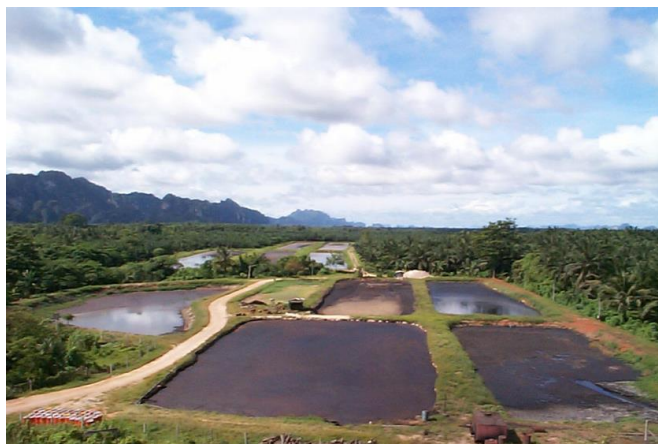
Figure 1.16 Conventional palm oil mill effluent treatment
