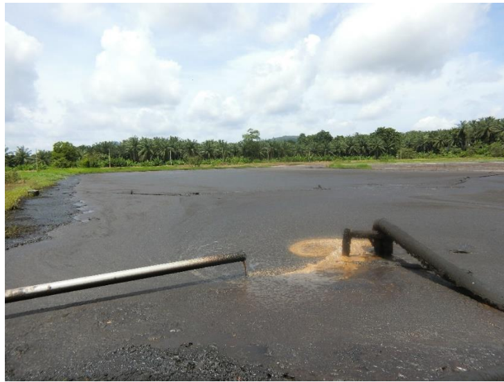
Figure 1.15 Raw palm oil mill effluent
