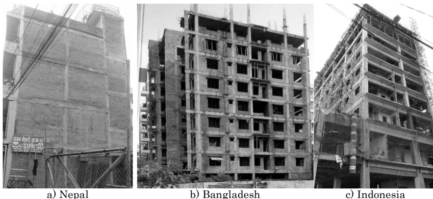
Photo 1 RC buildings with brick masonry infill walls
