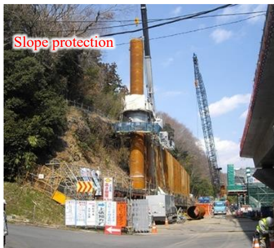
Figure 1.3 One of the constructed cantilever type steel tubular pile (CSTP) walls in Tokyo (Miyanohara et al., 2018)
