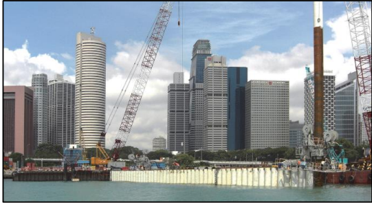
River revetment and highway protection wall (Singapore) Conservation of surrounding environment with no noise or vibration
