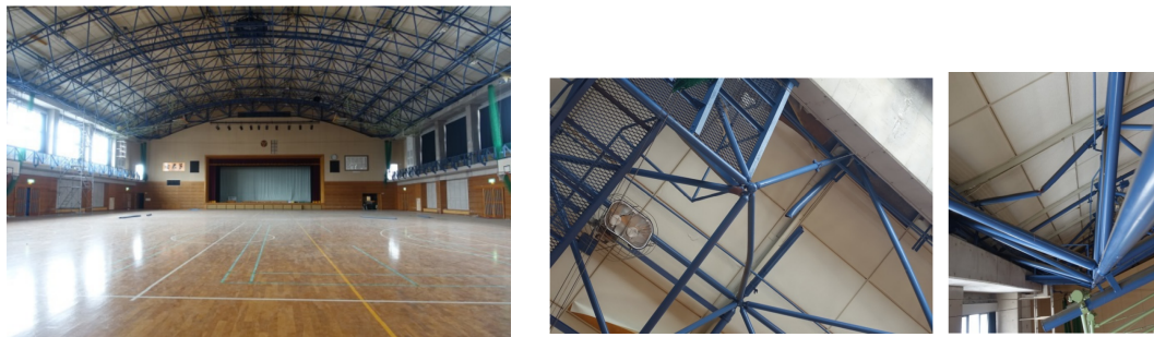
(a) Curved space truss roof
