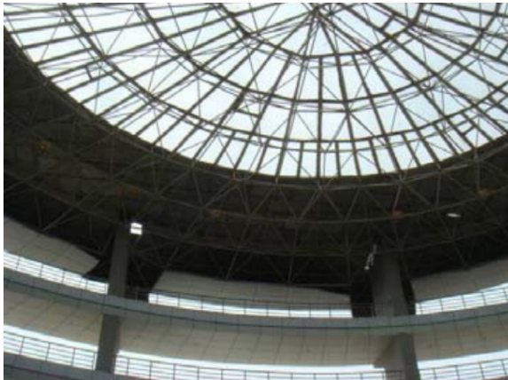
(a) Grid shell roof
