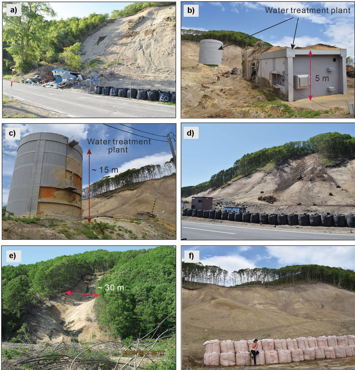
Fig. 5 Field survey photos of landslides following the September 2018 earthquake around the Atsuma area of Hokkaido (Japan). a A shallow landslide near a road. b, c A water treatment plant destroyed
