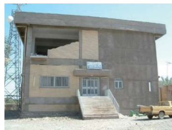
(a) the 2009 Sumatra earthquake (b) the 2003 Bam earthquake Fig. 16 Out-of-plane failure of masonry walls on upper floors of earthquake-damaged RC buildings
