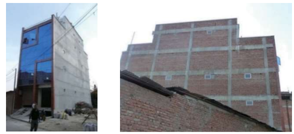
(a) North view (b) Southeast view Photo 1 Overview of the investigated building
