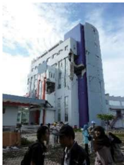
(a) the 2009 Sumatra earthquake (b) the 2003 Bam earthquake Fig. 16 Out-of-plane failure of masonry walls on upper floors of earthquake-damaged RC buildings
