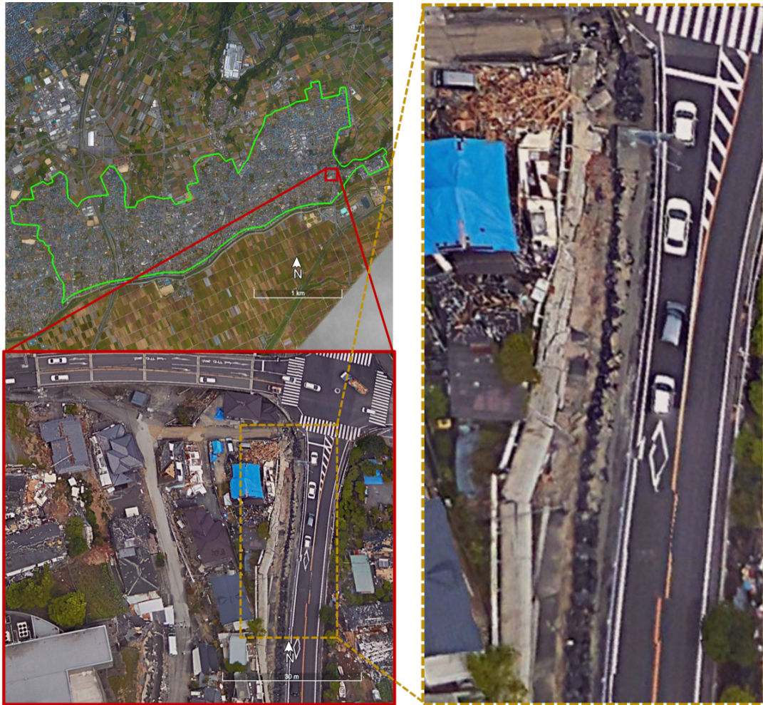
FIGURE 4.13: Overview of the area with large ground deformations. Green: the central area of Mashiki Town. Red: study area where large ground deformations occurred. Gold: Observable ground deformations in this area.
