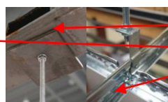
Photo.4 Boundary detail Photo.5 hanging bolt detail
