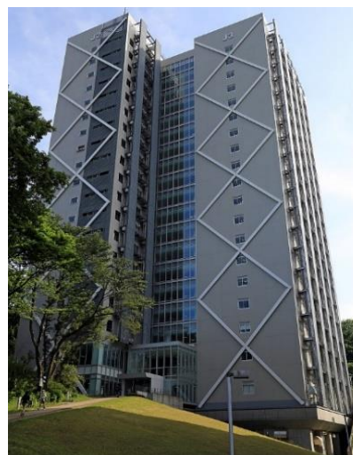
Fig.1 Photo of J2-3 building (Left: J2 building; Right: J3 building)
