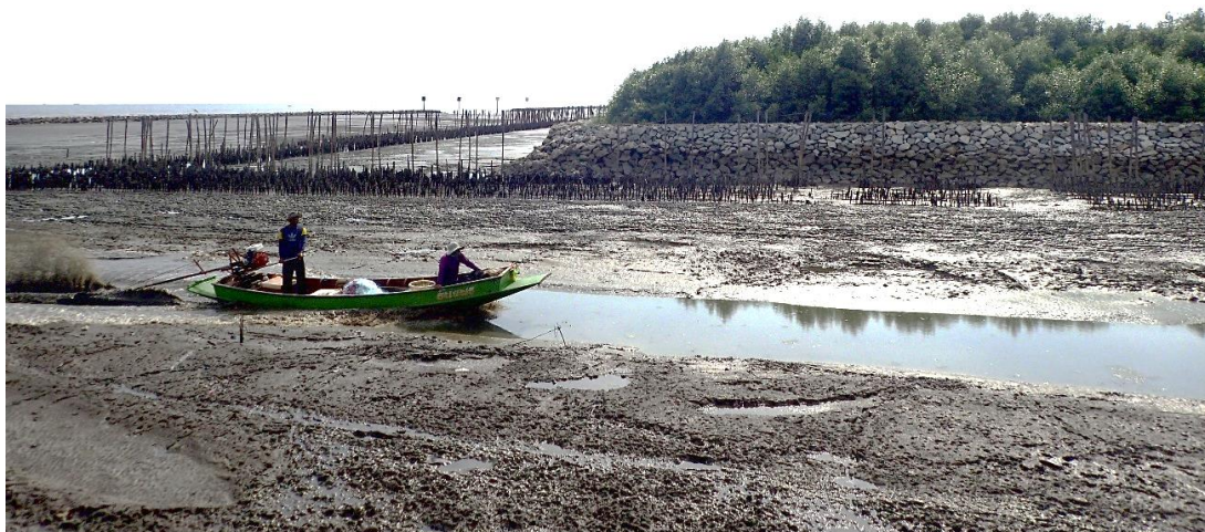
Figure 4. A successful mangrove plantation in Samut Prakan, Thailand. However, the rubble breakwater stopped the forest expansion. The mangroves were initially protected by bamboo breakwaters, but they were damaged by waves and no longer serve their purpose [photograph captured in May 2018 by the first author].
