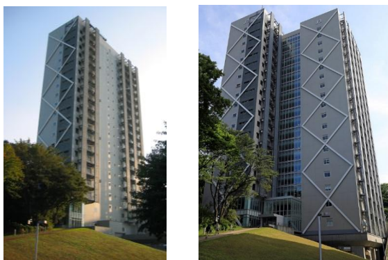
(a) J2 building
